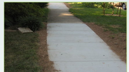
Completed sidewalk repair
