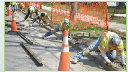
Concrete is smoothed and finished
